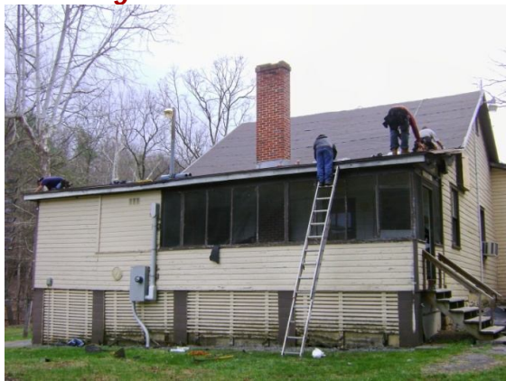
The Dining Hall's New Roof
