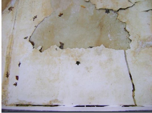
The Swimming Pool Before and During Repairs
