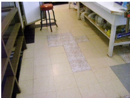
The Kitchen Floor – Old and New Floor
