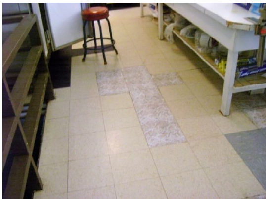
The Kitchen Floor – Old and New Floor
