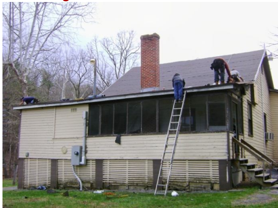
The Dining Hall's New Roof
