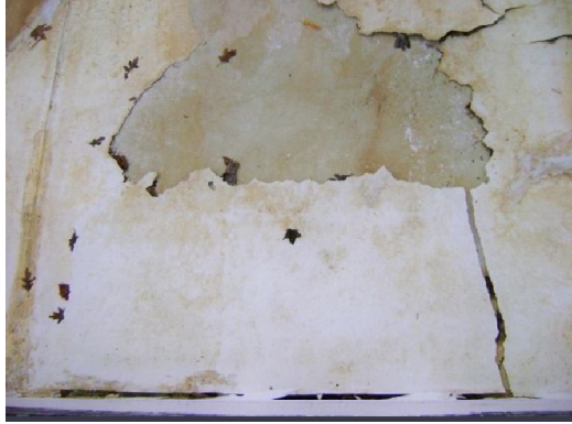
The Swimming Pool Before and During Repairs
